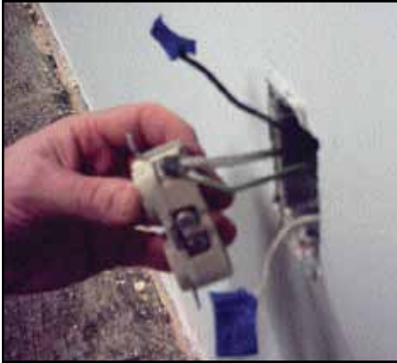
Figure 1. Use ground screw of electrical outlet connected to metal junction box and equipment ground for grounding.
